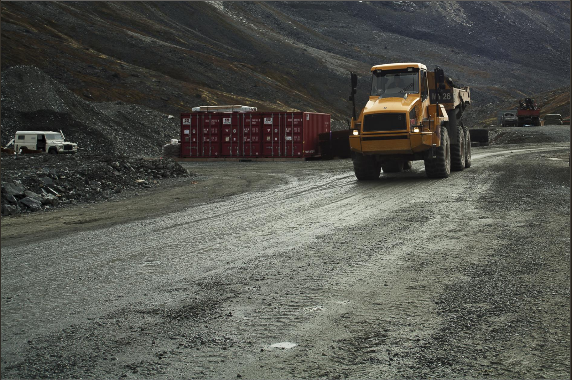
A truck transports the ore to the harbour, October 2006
