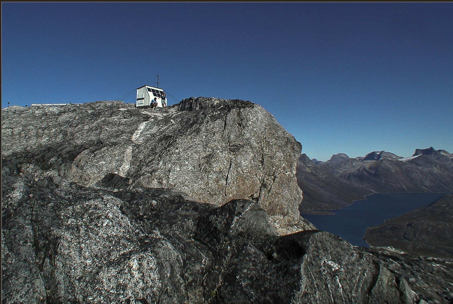
Communication link at the top of the mountain Store Malene, August 2003
