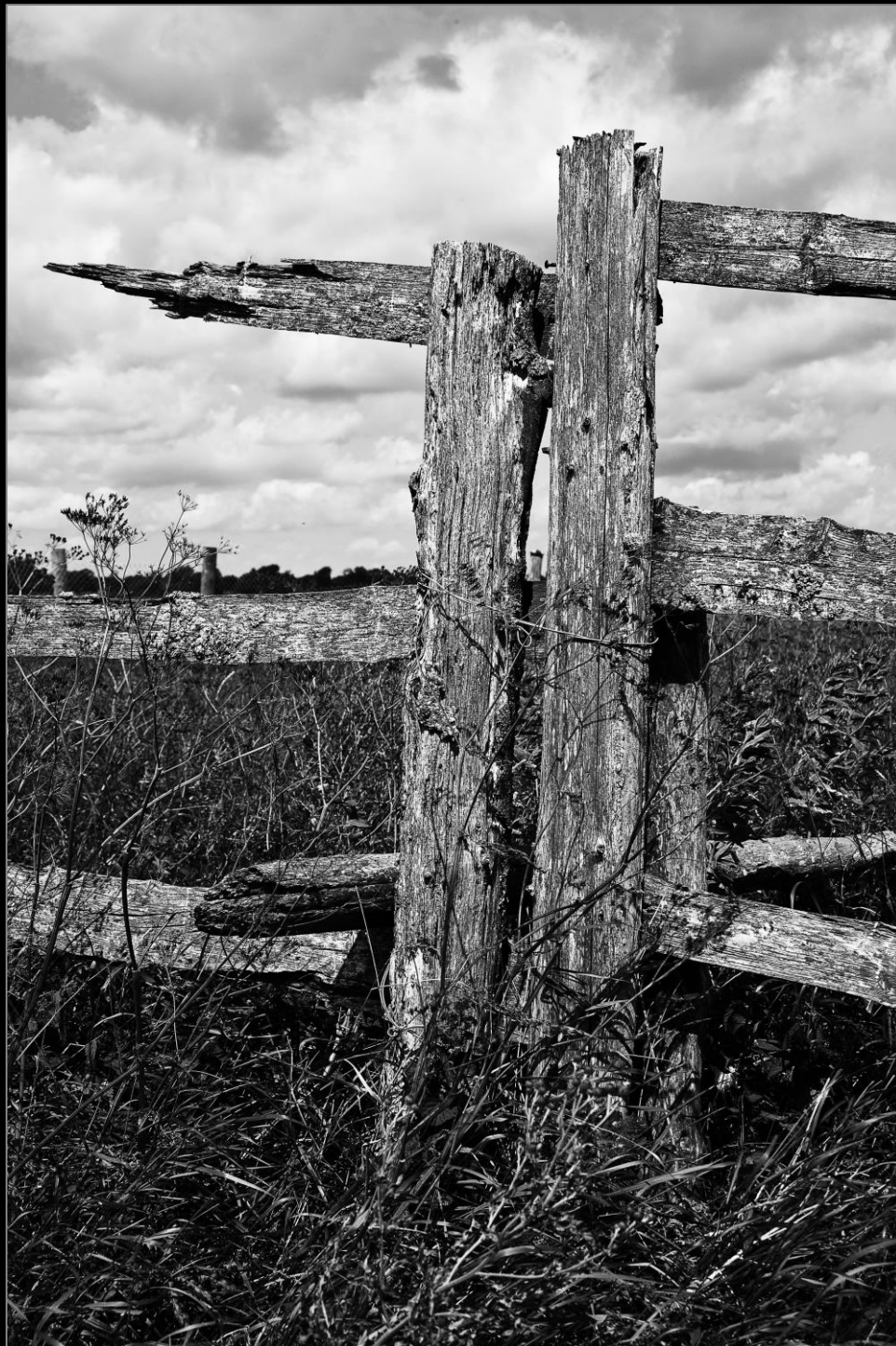
Grønnevej, Lille Vildmose, Himmerland in Denmark, July 2013
