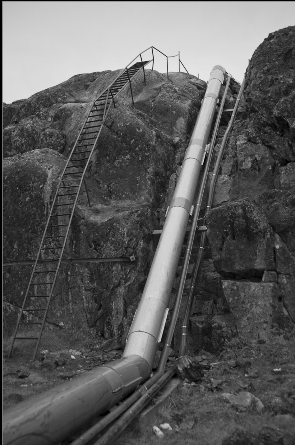
The water pipe to the centre of Nuuk, September 2007
